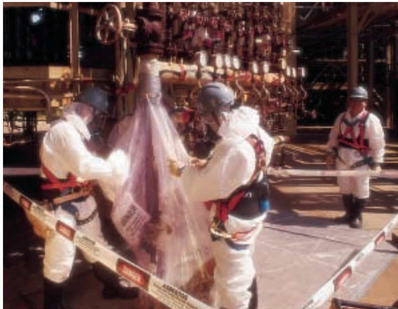
Figure 11.12 Asbestos was formerly used to insulate buildings. It is now known to cause lung cancer and other lung diseases and must be removed from these buildings, as shown here.
