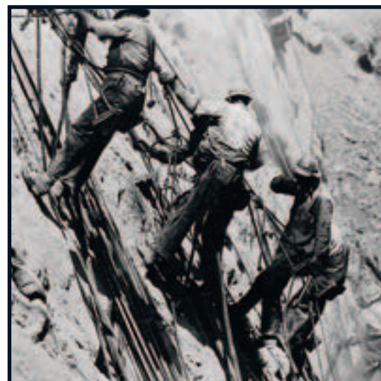
Suspended on ropes, “high scalers” armed with dynamite and jackhammers prepare the walls of Black Canyon to take the concrete of Hoover Dam. Such work was hazardous. Twenty-four workers fell to their deaths during construction of the dam.
