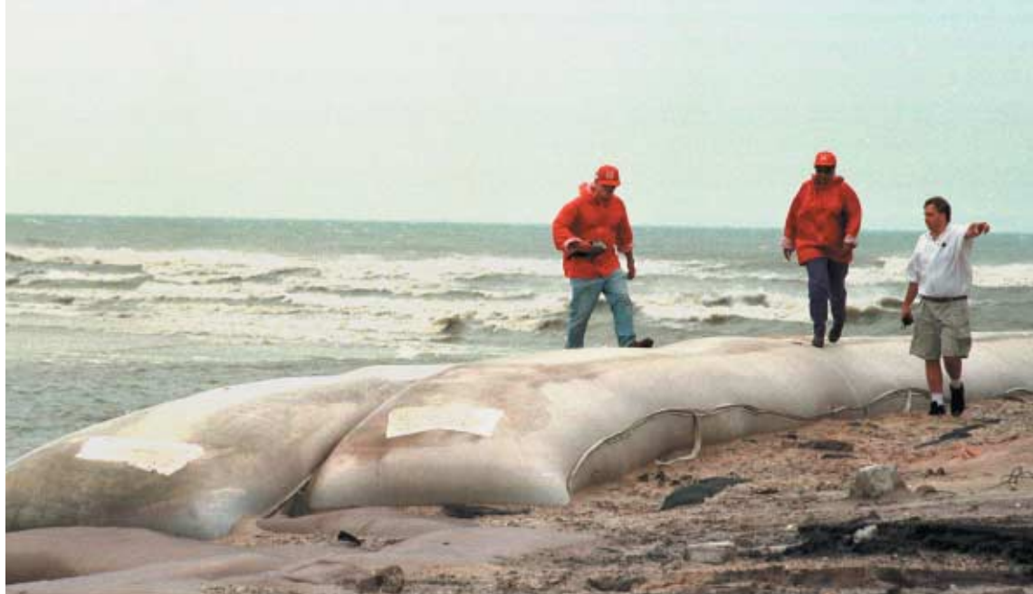
Figure 4 ► Engineers inspect beach erosion caused by hurricane Bonnie, which struck Wrightsville Beach, North Carolina.
