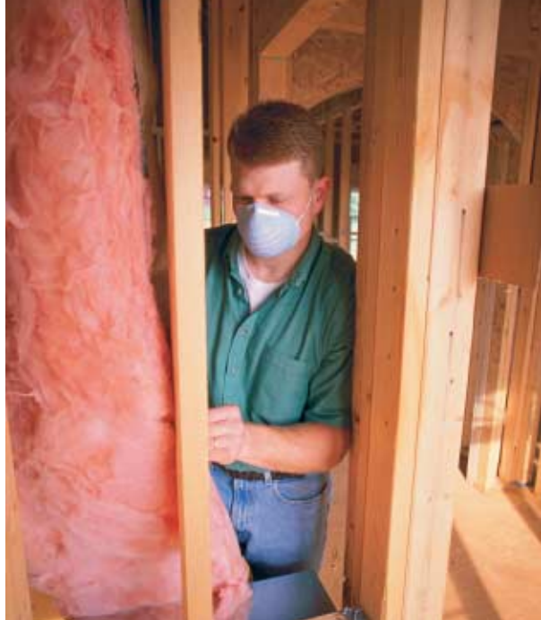
Figure 4 ► Fiberglass insulation is used in homes to reduce the energy required for heating and cooling.
