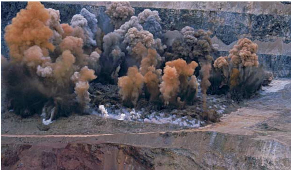
Figure 1 ▶ The surface of this gold mine in Nevada is being blasted to remove layers of rock.
