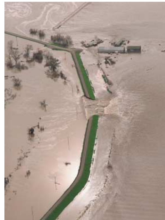
Figure 3 ► Week-long storms in Modesto, California, in 1997 broke this levee and caused flooding.
