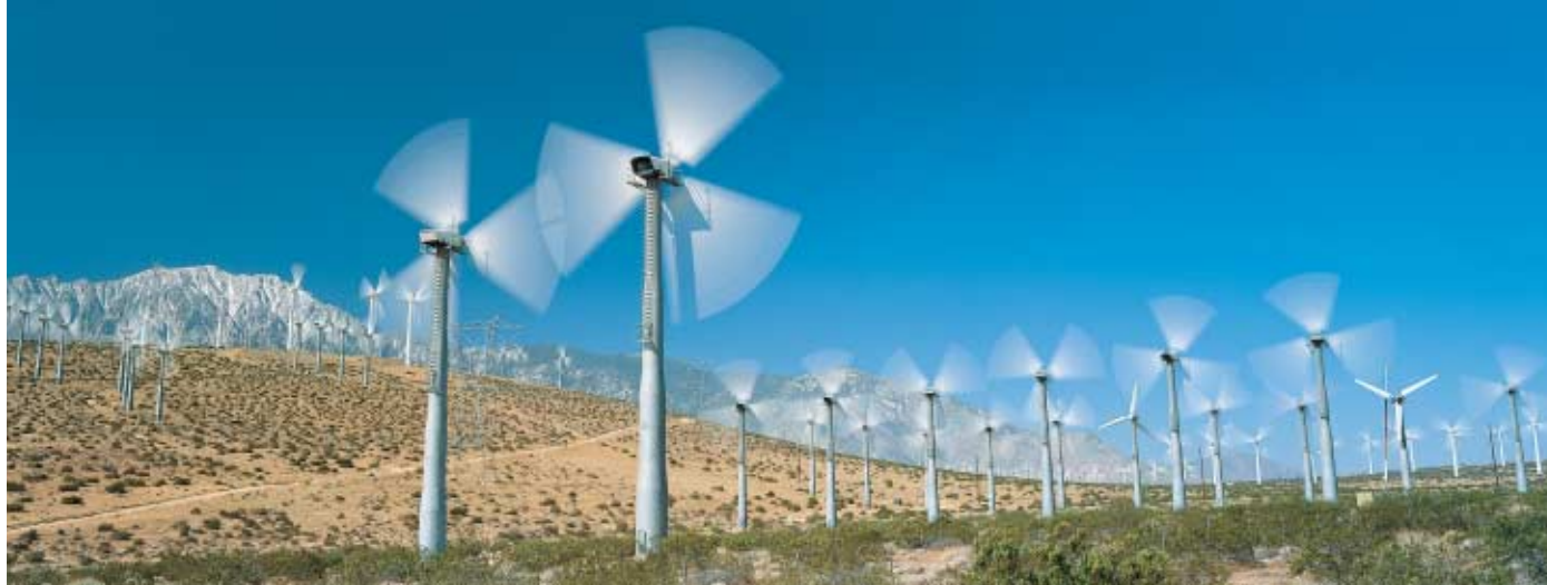
Figure 3 ▶ The spinning blades of a windmill are connected to a generator. When winds cause the blades to spin faster, the generator produces more energy.
