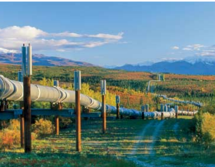
Figure 8 ► The Alaskan pipeline has carried more than 13 billion barrels of oil since it was built in 1977. The pipeline has also sparked controversy about the potential dangers to nearby Alaskan wildlife.
