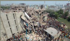
A collapsed garment factory in Savar, Bangladesh. Source: AP
