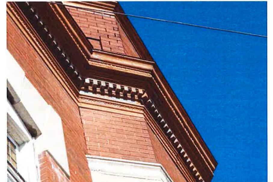
Dentil sheet metal cornice at corner turret at 224 N. Harrison. (Top)
