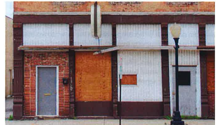
Although in disrepair, the original storefront proportions and cast iron pilaster remain at 116 N. Harrison - the former Happy Times bar.
