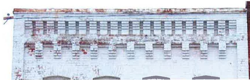
Brick detail at cornice on W. Washington
