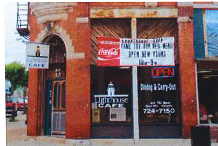
Historic storefront remains with minor alterations. Decorative cast iron column and beam detail remains. Visual clutter is created by various signs and banners.
