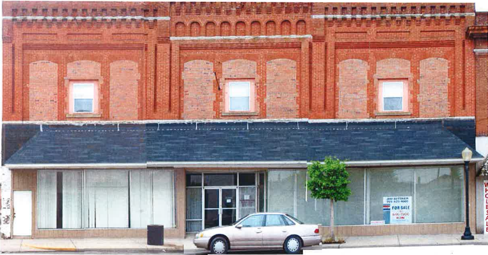
Corbelling and brick and stone arch detailing at center bay. (Right)
