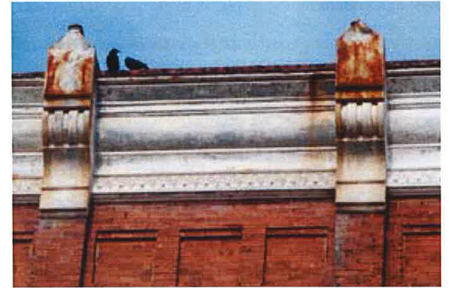
Multi-profiled, intricately detailed metal cornice in deteriorated condition
