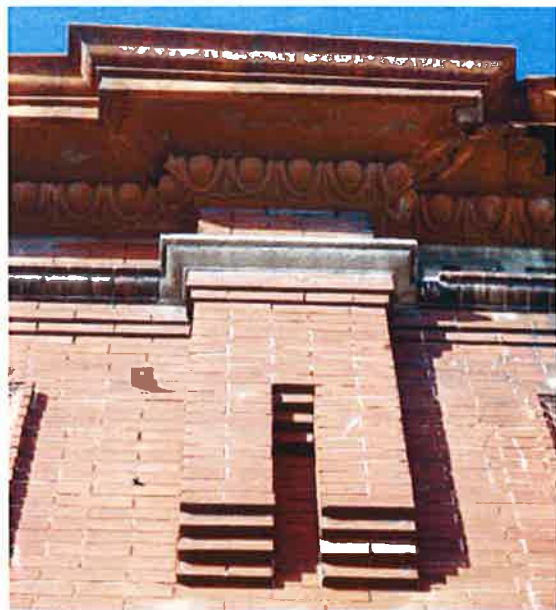
Egg and dart detailing at metal cornice and decorative masonry at 220-222 N. Harrison
