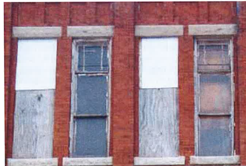
Boarded and deteriorated windows with original double hung and divided-lite transoms
