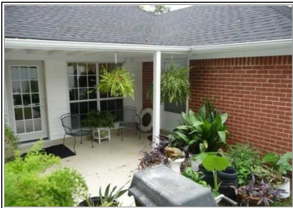
REAR OF SUBJECT PROPERTY
