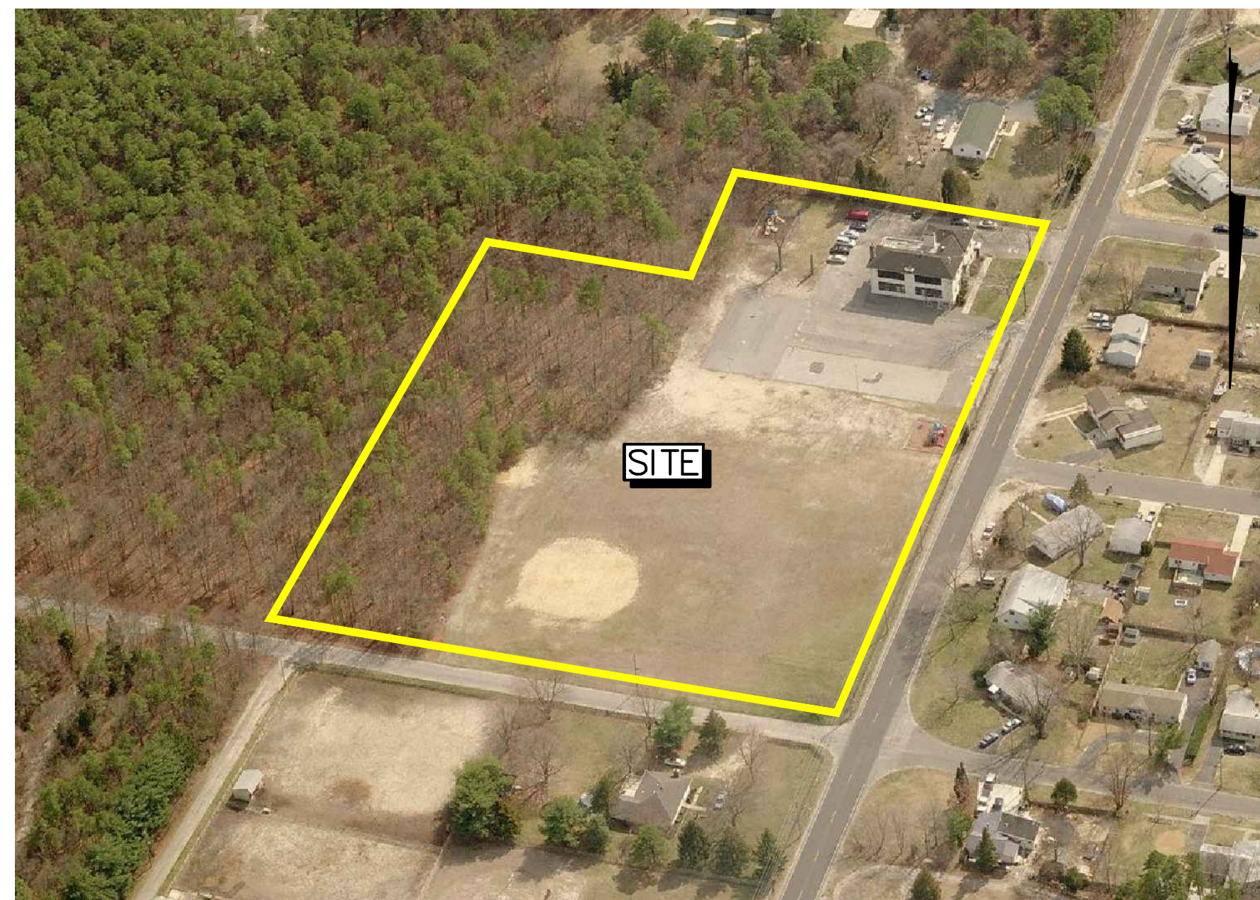
SITE PHOTO FACING SOUTH
