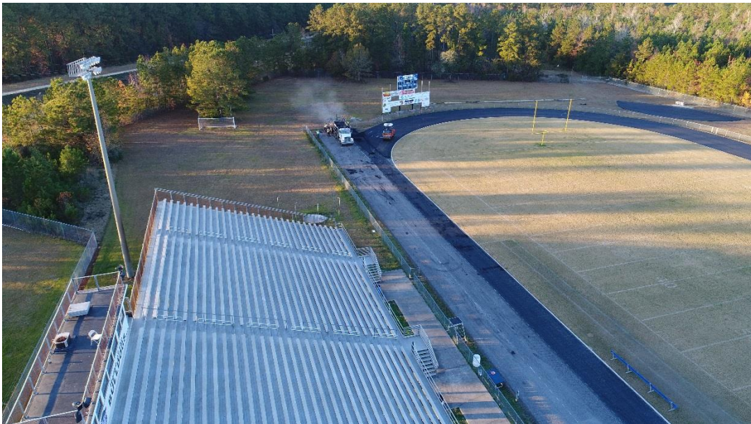
Paving operations on November 29, 2017
