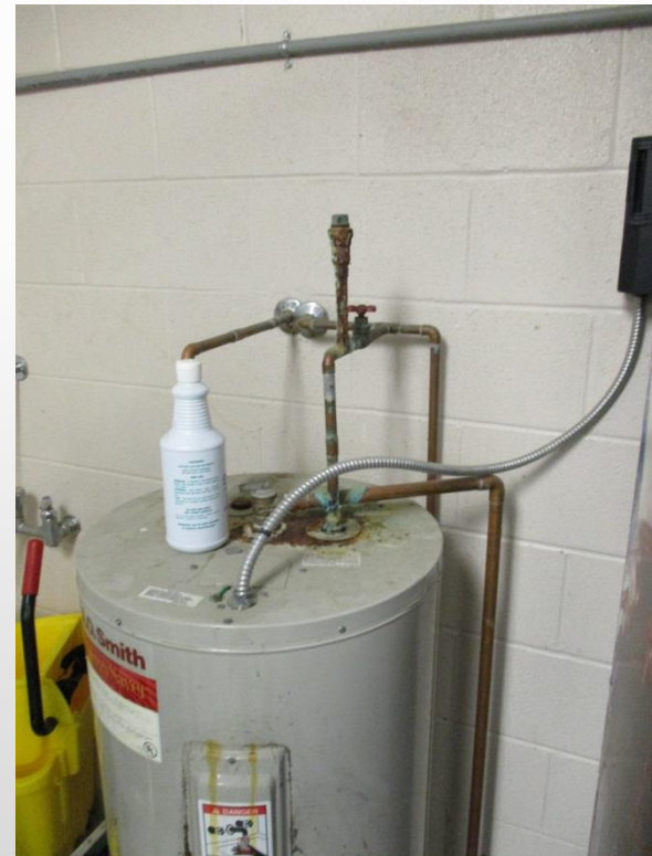
Hot Water Heater Replacement Several Schools
