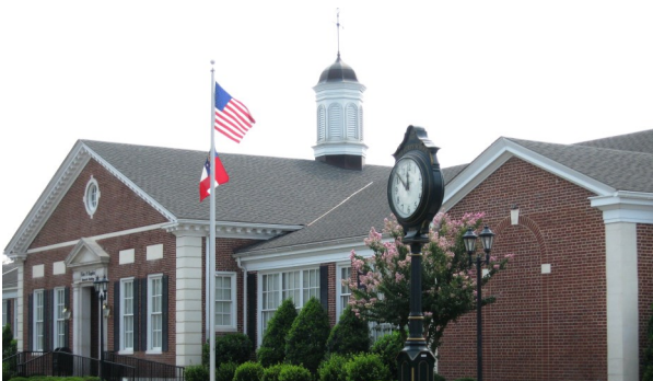
Eric P. Staples Building, Central Office, Perry, Georgia
