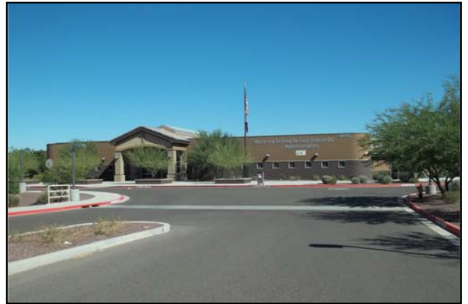
Picture 2 – District Office Complex.
