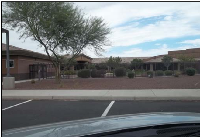
Picture 3 – North view of District Office Complex.
