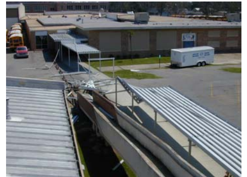
The canopies at Moss Point High School crumbled during the storm.
