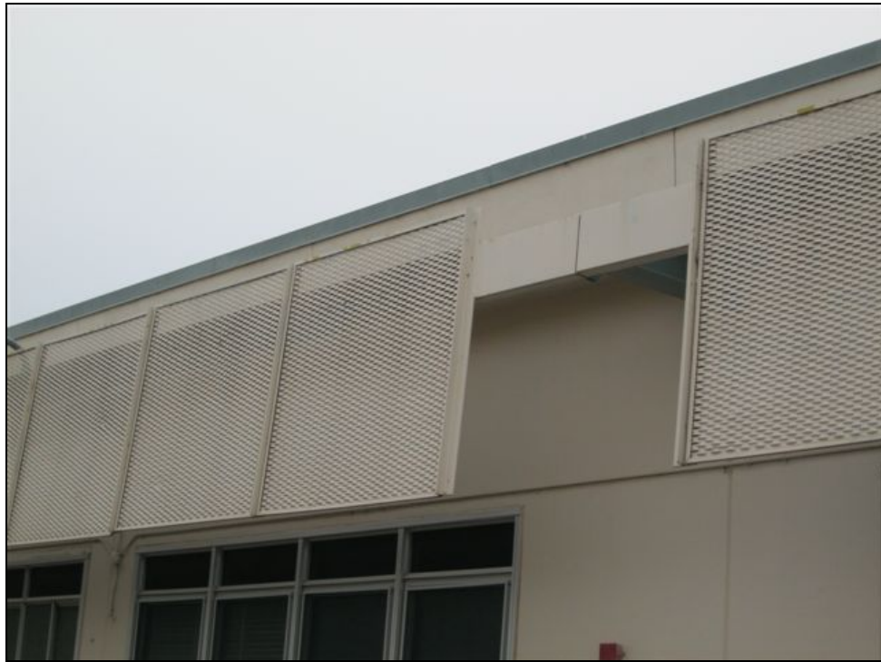
ERHS Gym - Removing Sun Screens to Update the Look
