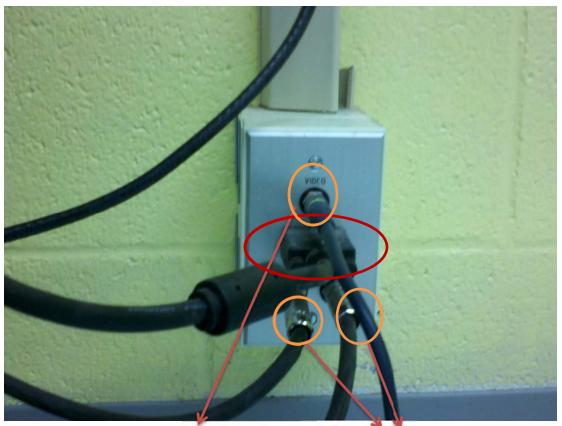
Also on the wall outlet is the video plug on top and the two speaker wires . The video plug should be coming from your VCR or DVD player. The speaker wires will be coming from the Amplifier (see next picture).
